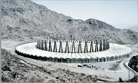
Muna Reservoir, Saudi Arabia "A cable-stayed bridgelike roof structure"
