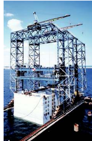
Gabes Port, 3000 ton Caisson Launching, Tunisia
