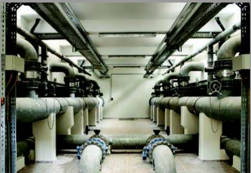
Sirt Sewerage Treatment Plant, Rapid Sand Filter, Turkey
