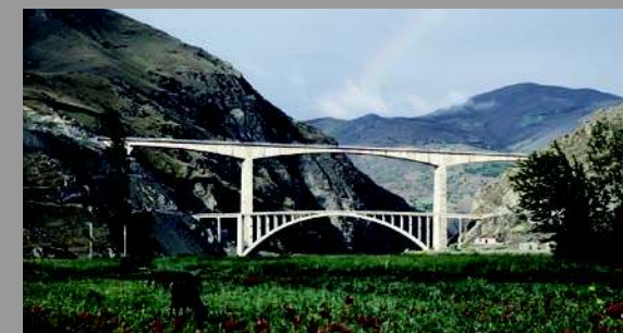
Kömürhan Bridge, Turkey "First bridge built with free cantilever method in Turkey"
