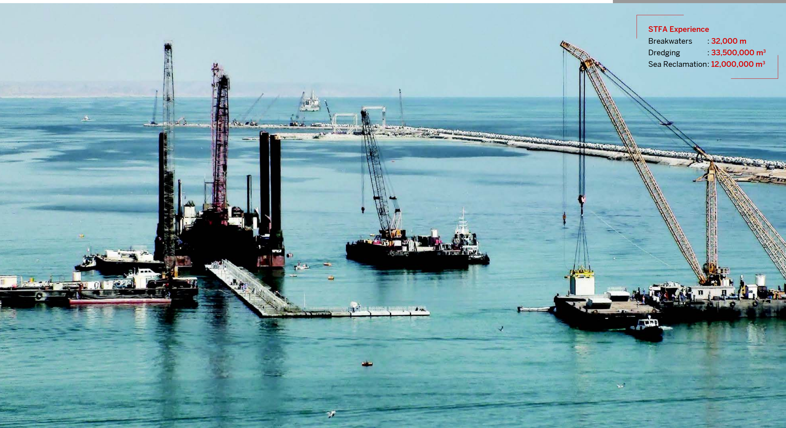
Gabes Port, 3000 ton Caisson Launching, Tunisia
